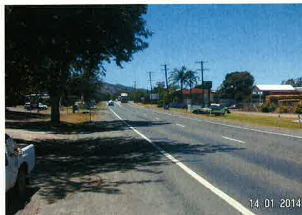
Plate 4. Easterly view of the New England Highway Nemingha.
